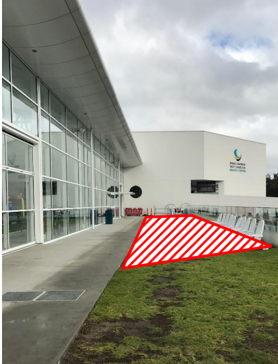
Figure 4. Grassed area for temporary storage of materials.
