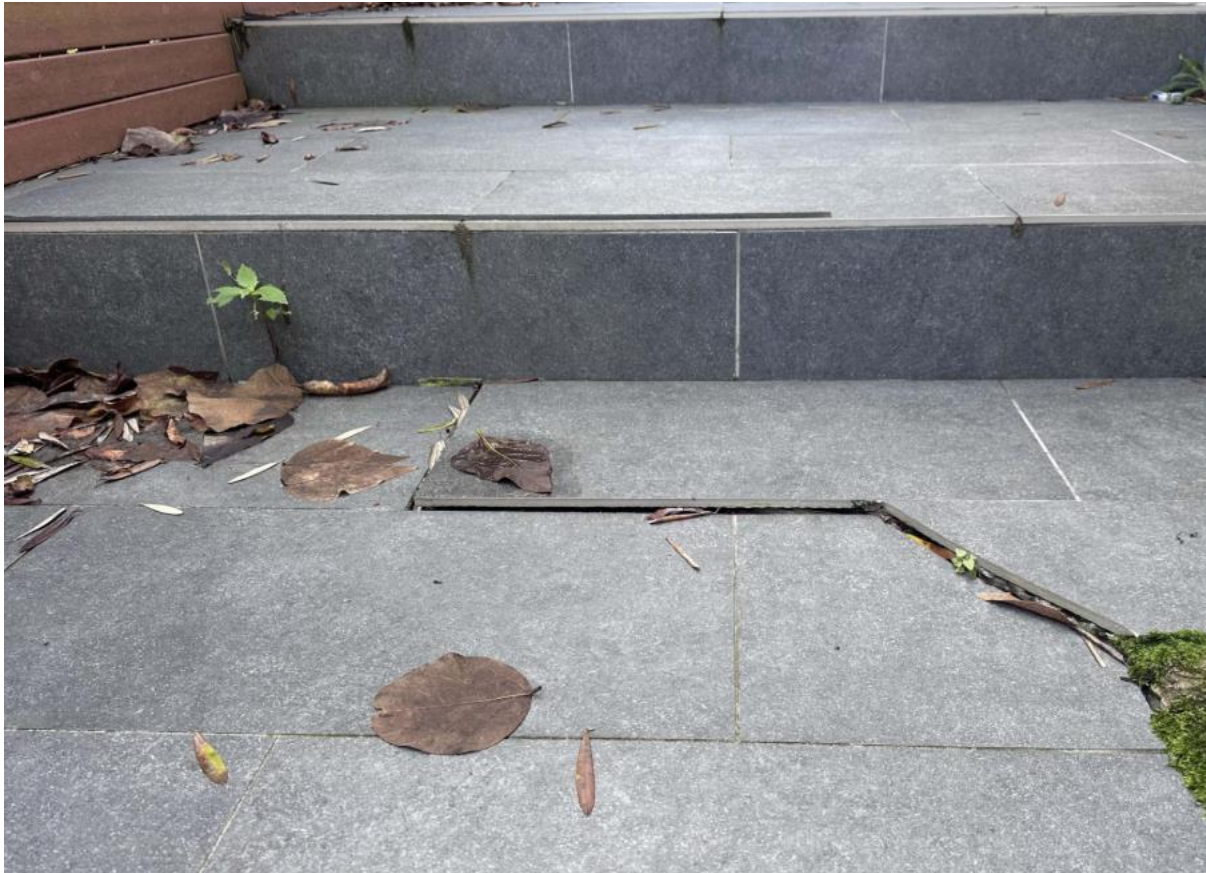
Figure 1 – Photos of land movement at 5A Cooleena Road – immediate adjacent to indicative dwelling proposed.
