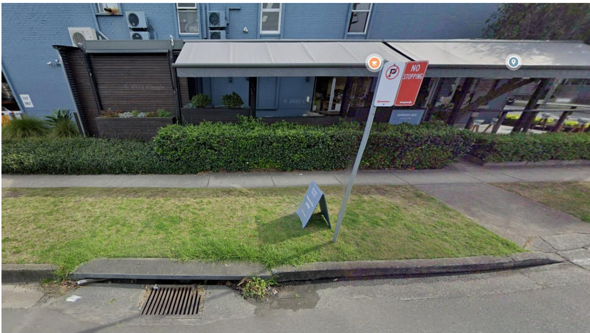
Stormwater pit in Roseberry Street (Google Street View)
