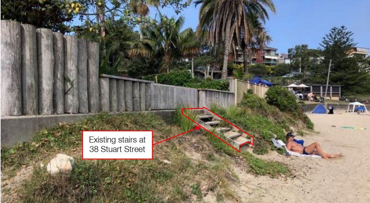
Figure 2: Existing stairs at the rear of 38 Stuart Street, Manly
