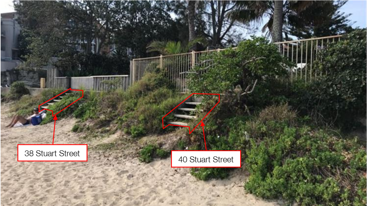
Figure 3: Existing stairs at the rear of 40 Stuart Street in the foreground and existing stairs at rear of 38 Stuart Street, Manly in the background
