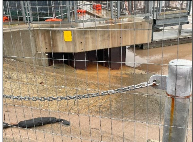
Figure 2 – Sheet pile along the sea wall
