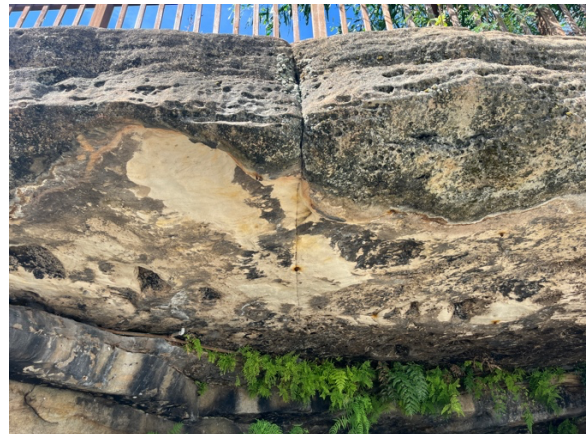
Photo 4: Example of fine vertical jointing in the over hanging bedrock
