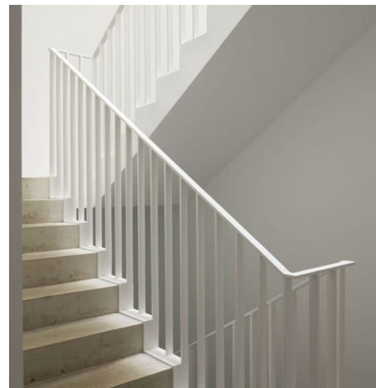
White painted steel internal balustrade
