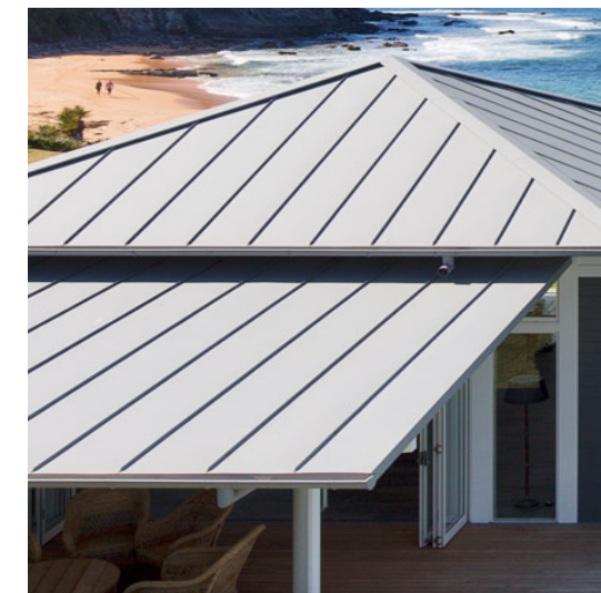
Standing Seam Metal roof cladding
