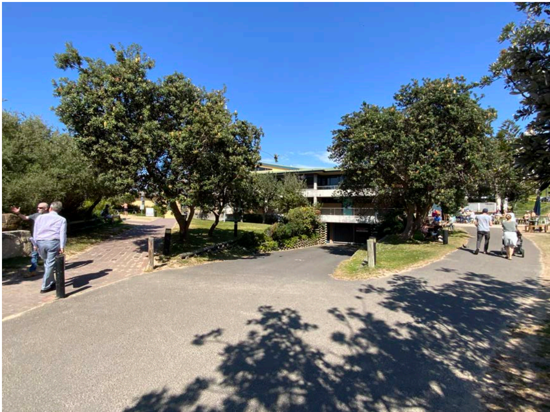
Figure 15: View of the 1987 additions
