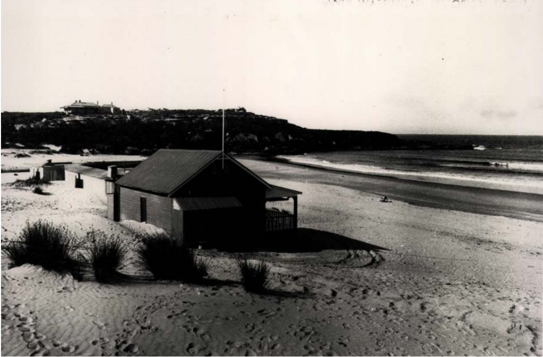
Figure 28: View of the first Freshwater Surf Life Saving Club building following the additions in December 1914. [Source: Northern Beaches Council Library Service. 'History Hub' Image No.47601]
