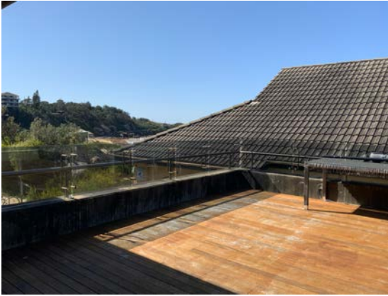
Figure 9: View of the roof terrace area of the 1987 additions.
