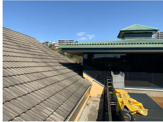
Figure 10: View of the contrasting roof forms.
