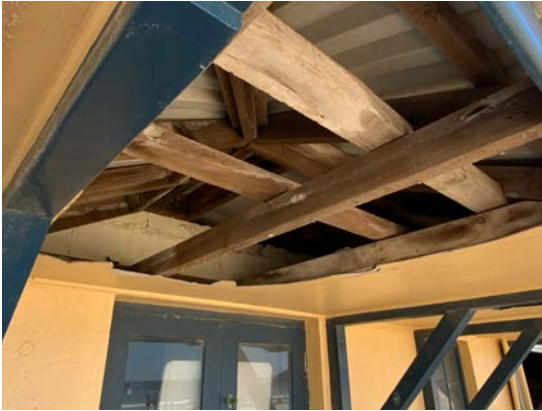
Figure 6: View of awning detail to beachside elevation.
