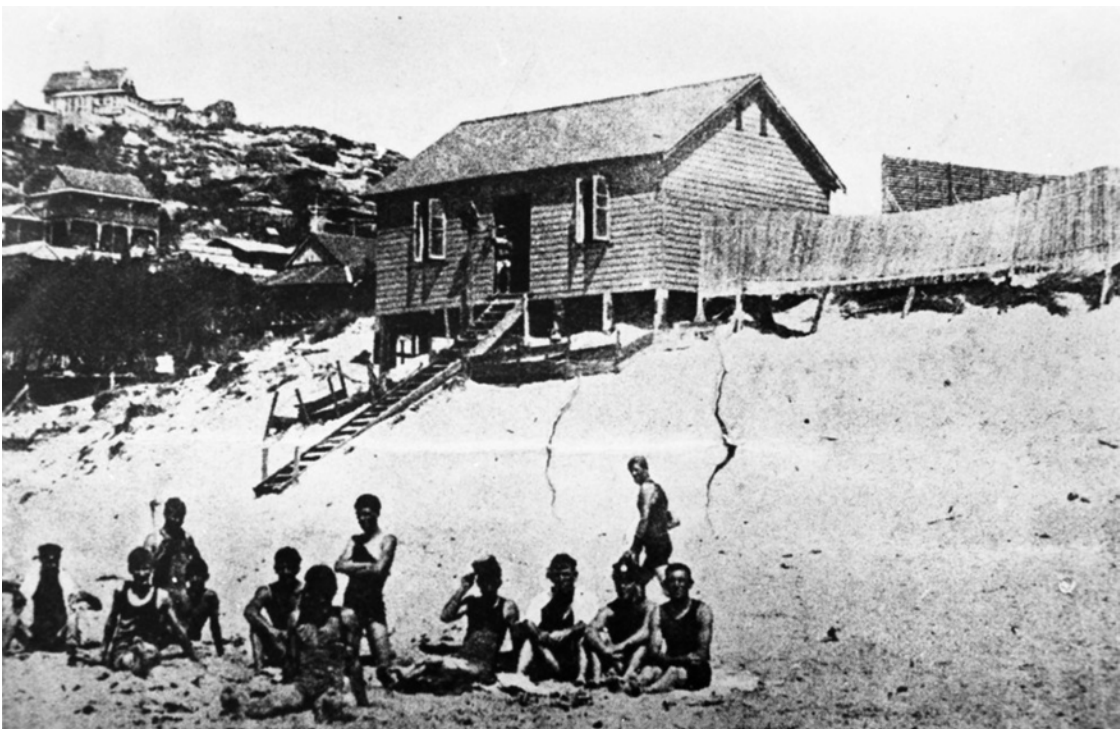
Figure 27: View of the first clubhouse c1913 following damage by high seas. Note much of the sand has been washed away, undermining the foundations of the building and fence. [Source: Northern Beaches Council Library Service. 'History Hub' Image No.42633]
