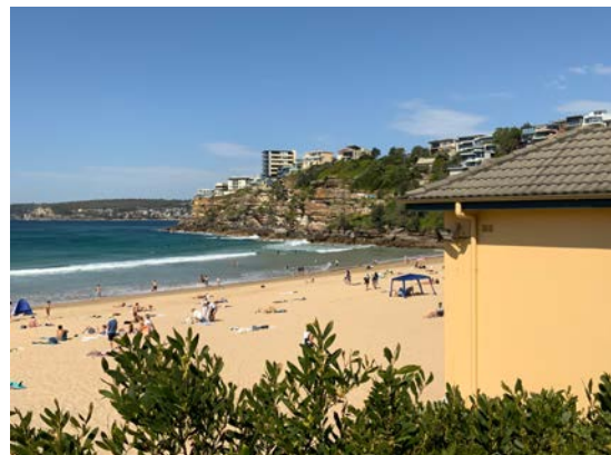
Figure 17: View of the original 1934 building at the beach.
