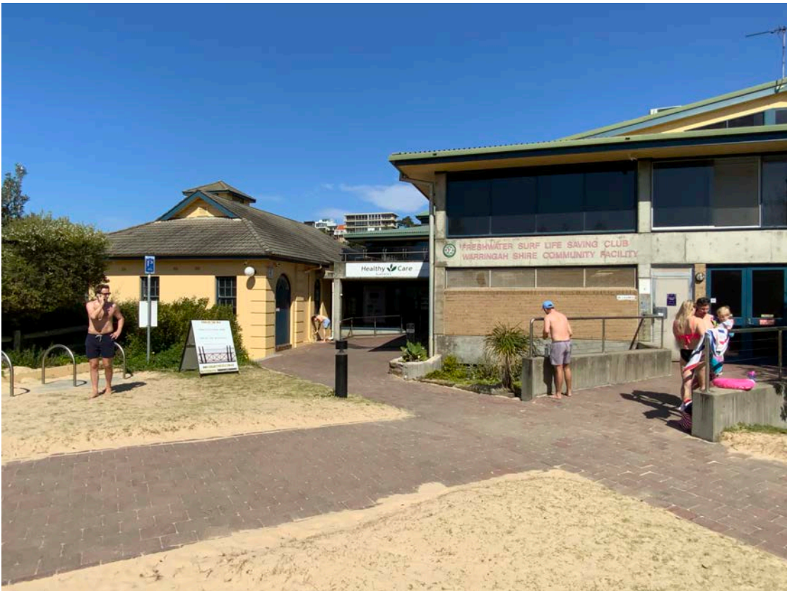
Figure 8: View of the northern side elevation.
