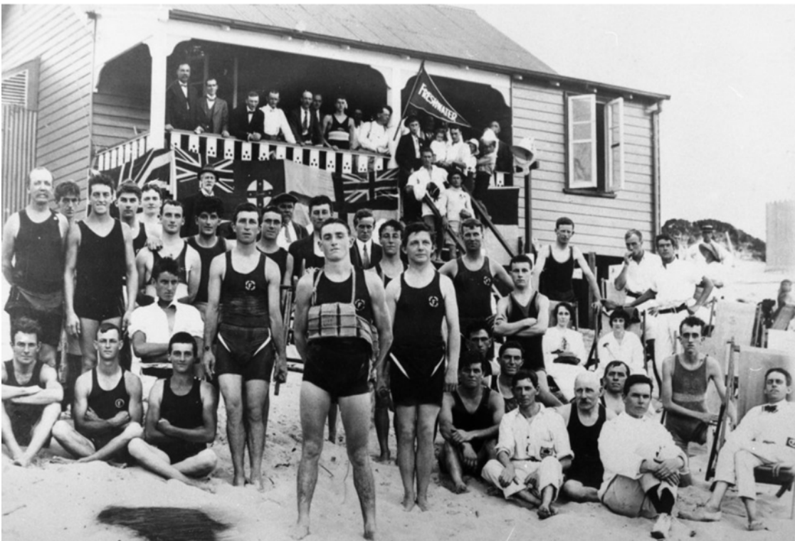
Figure 29: View of the extended Freshwater Surf Life Saving Club building following additions in December 1914. [Source: Northern Beaches Council Library Service. 'History Hub' Image No.42623]
