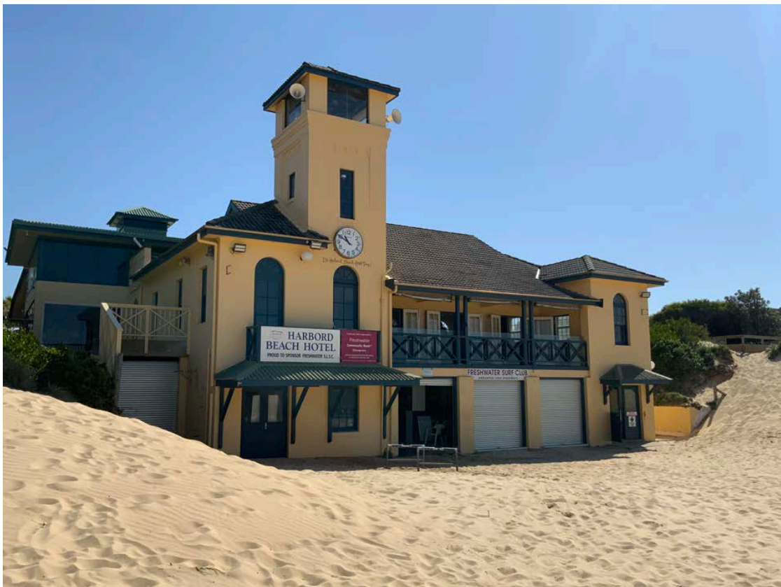
Figure 3: View of the Freshwater SLSC building as viewed from the beachside.
