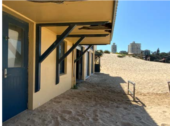
Figure 7: View of the beachside entry to the boatsheds.
