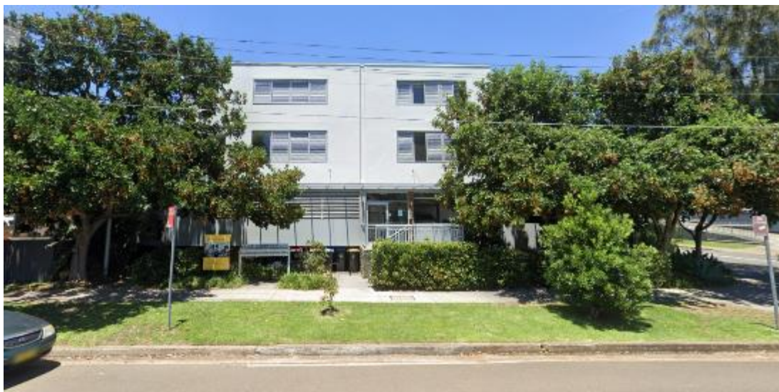
Figure 4: 3 storey shop top housing development at 9-11 Gondola Road
