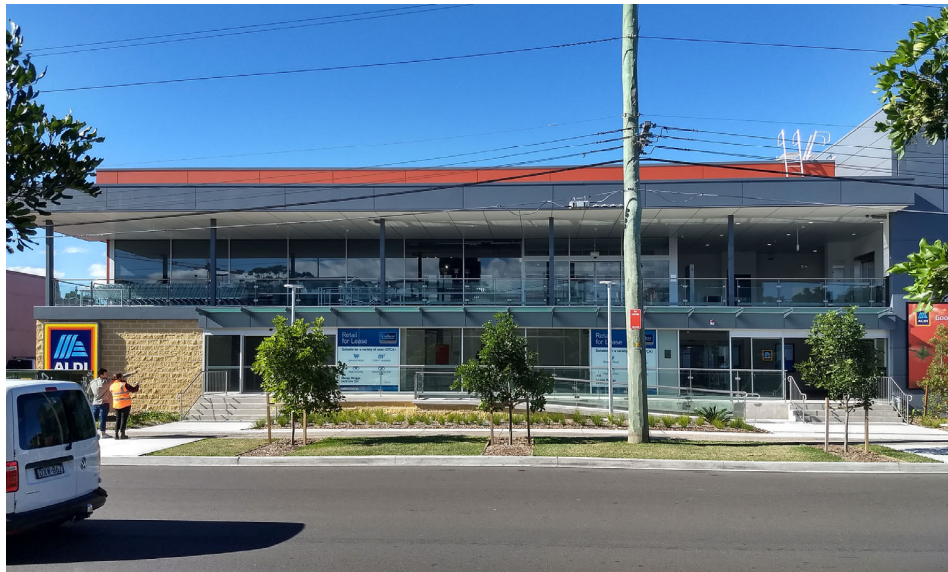
02 - View from across Roseberry st
