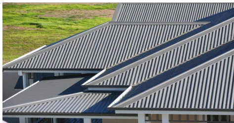
COLOURBOND METAL ROOF SHEETING POWDERCOAT FINISH 'IRONSTONE' OR SIMILAR WHERE MARKED ON ELEVATION.
