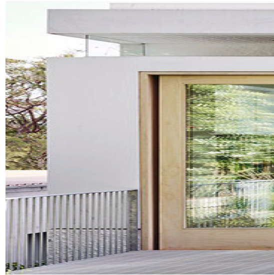
DOORS AND WINDOWS TIMBER
