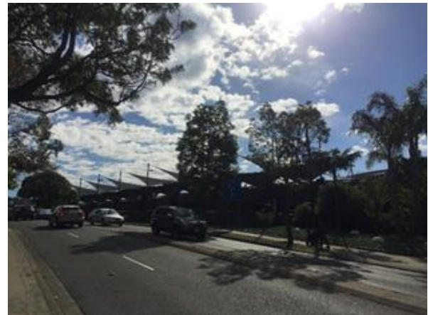
Picture 2 View of Car Park from Old Pittwater Road Source: Urbis
