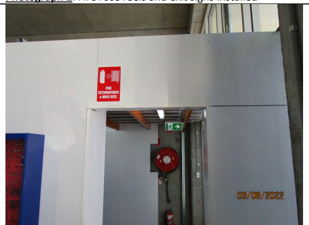
Photograph 4: Exit direction sign required above opening to reception area
