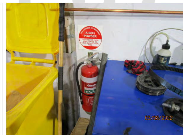
Photograph 1: Portable fire extinguishers installed
