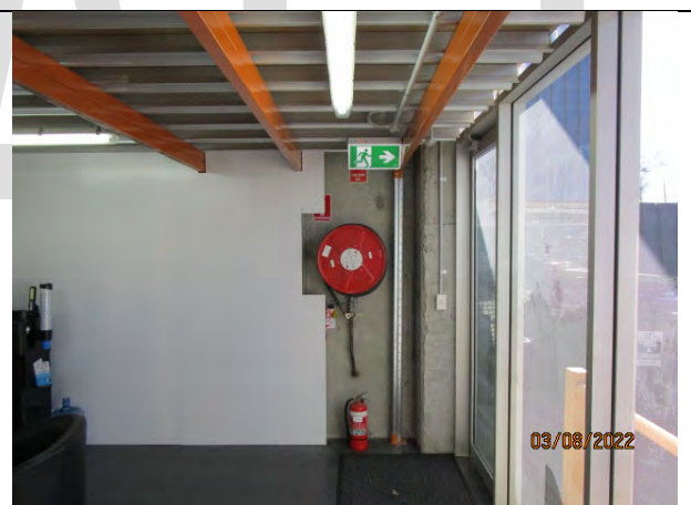
Photograph 2: Fire rose reels and exit signs installed
