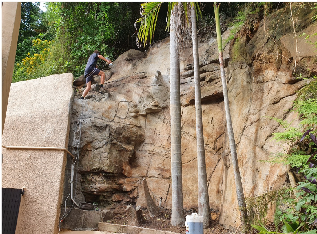
Proposed finishes on retaining with Mock Rock which painted to blend in with the natural landscape
