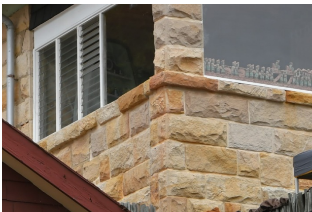
Irregular sandstone walls
