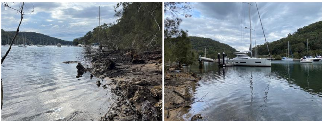
Figure 5: Waterfront structures to the (a) northeast and (b) southwest of the Subject Site.
