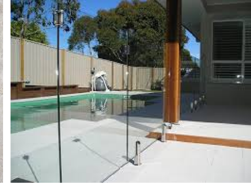
GLASS BALUSTRADES - 1.2M H - ENSURE NON CLIMBABLE AND COMPLIANCE WITH AS1926.1-2012
