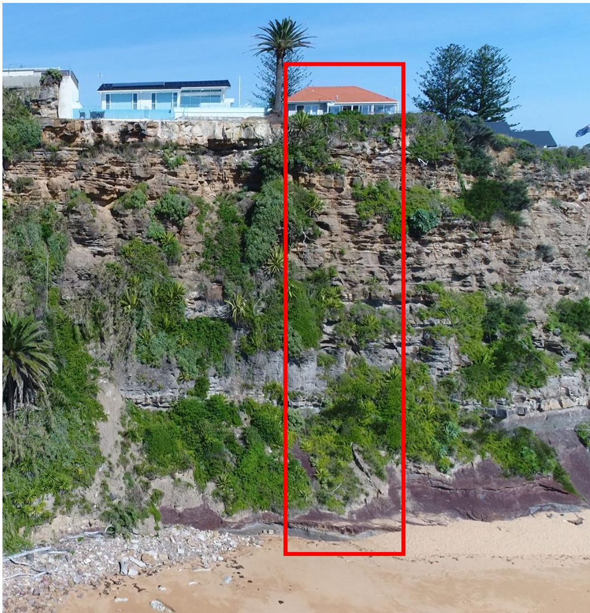
Photo 5 – approximate portion of cliff within property boundaries in red
