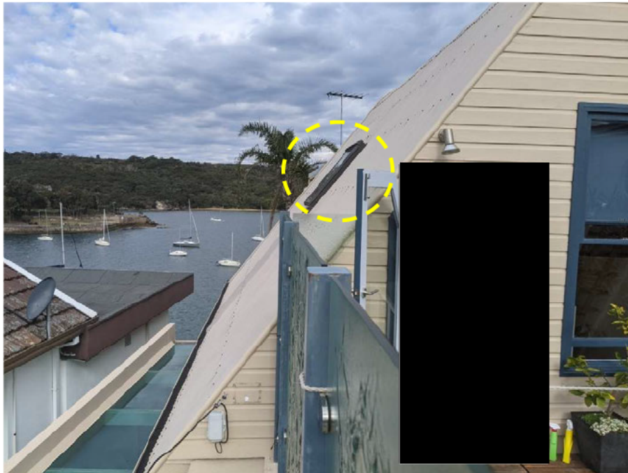
Figure 1: South view between 14-16 Addison Rd (prior to demolition) and skylight shown
