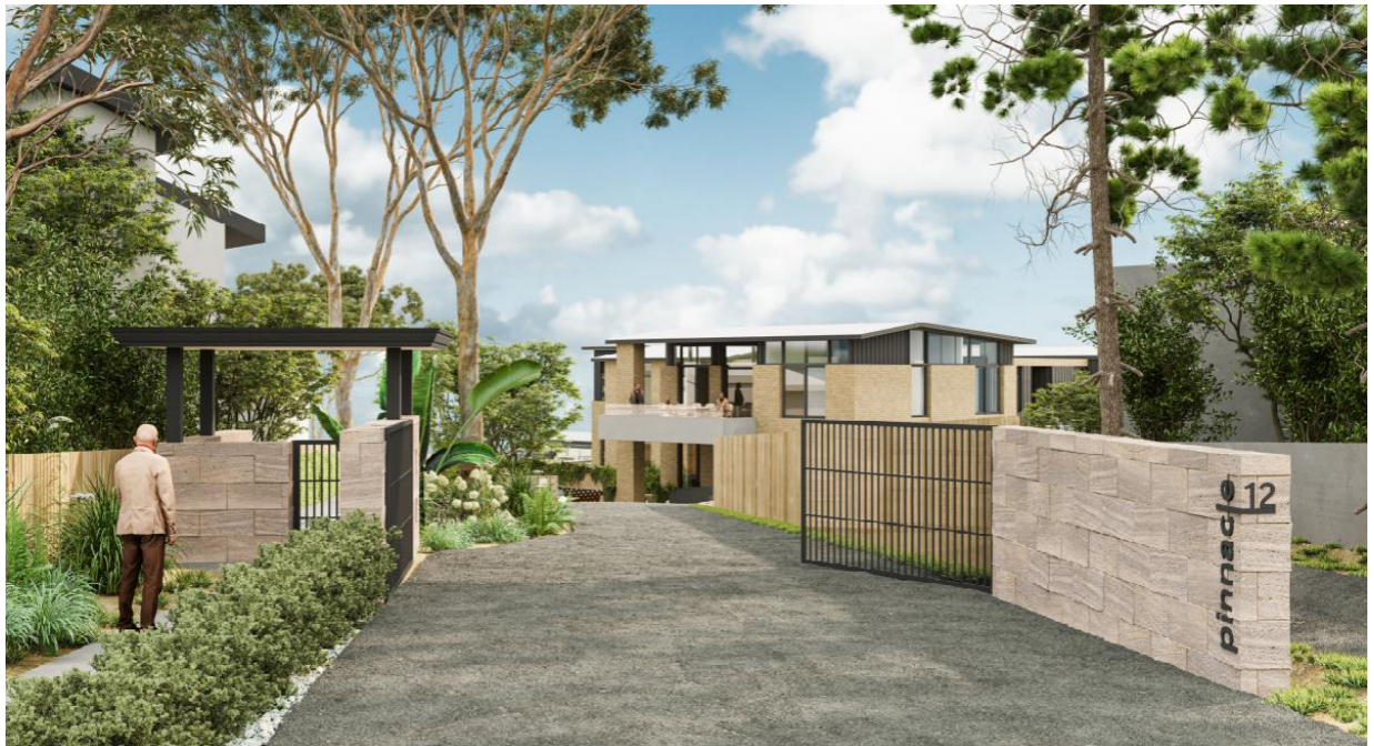
Figure 3 – Perspective image of the development as viewed from Gladys Avenue depicting a two storey built form as viewed down the driveway alignment. Note the breaching elements will not be discernible as viewed from the street.
