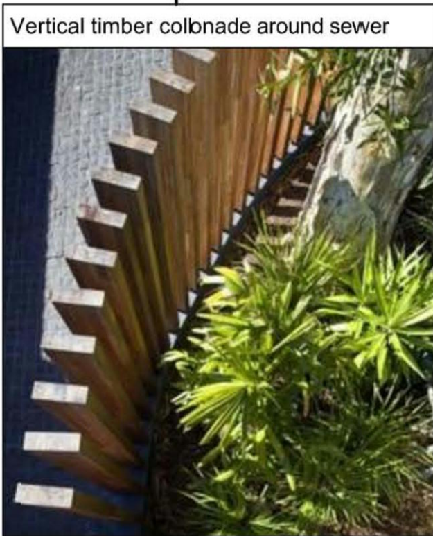
Vertical timber colonnade around sewer
