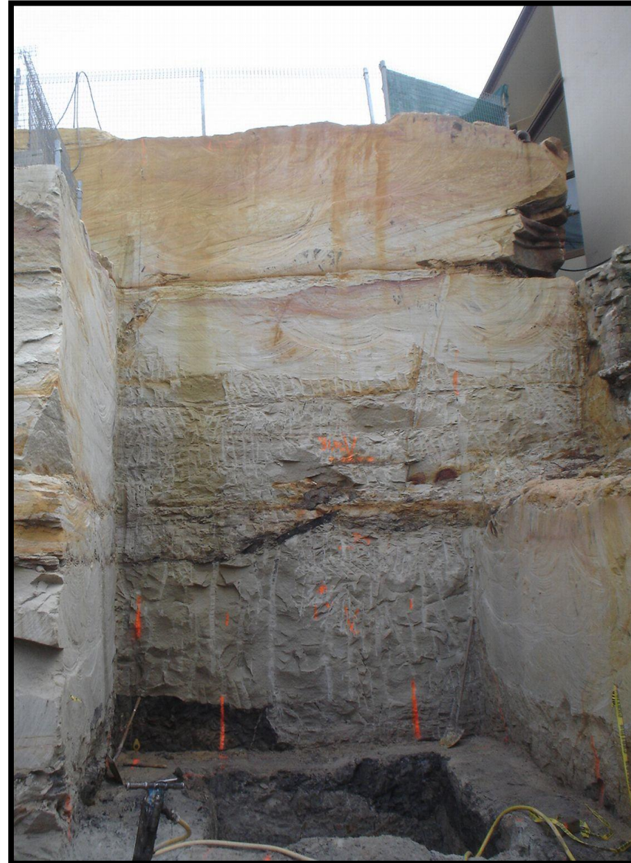
Rear, north-eastern corner of basement excavation, looking north
