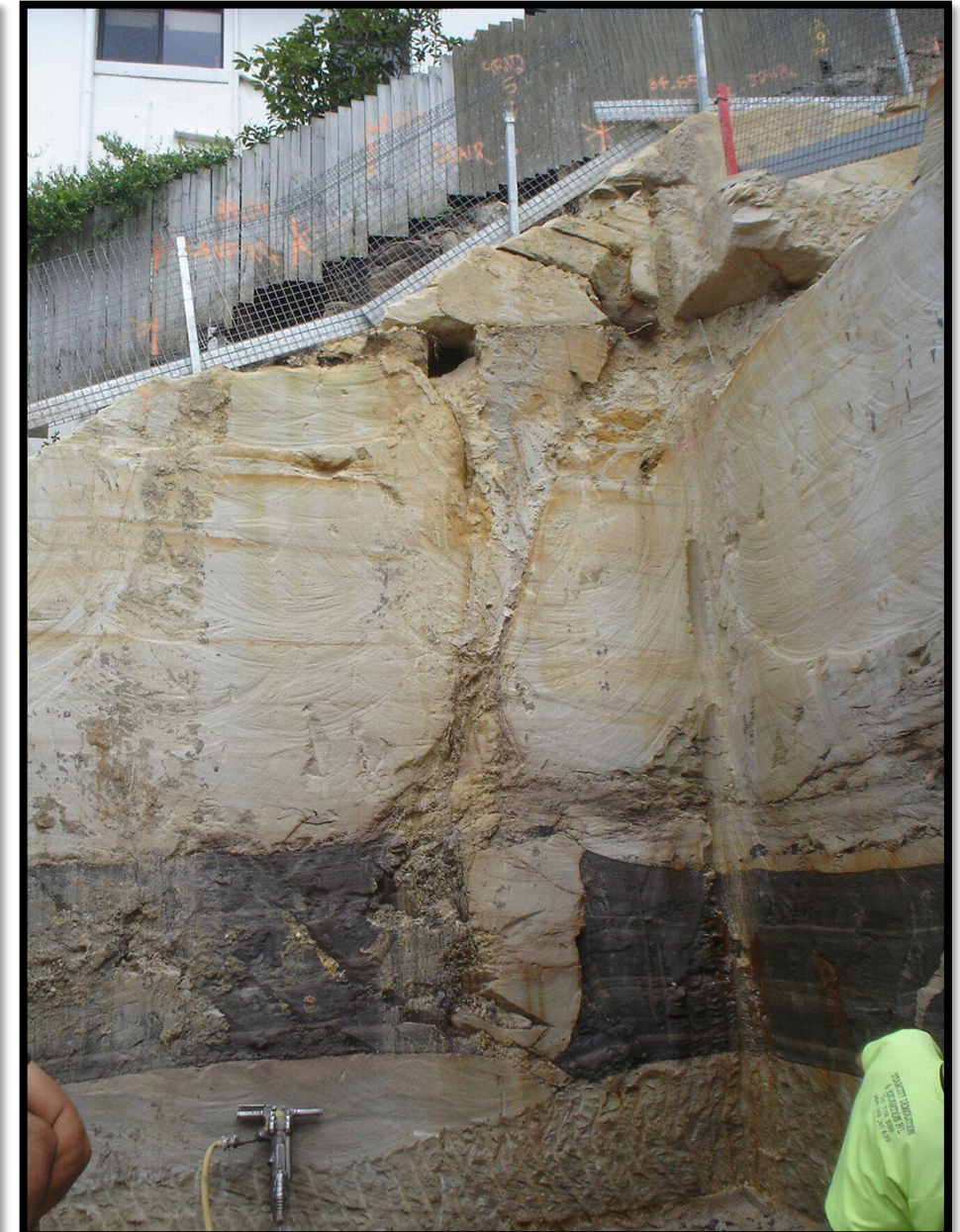
Rear north-western corner of basement excavation, looking west
