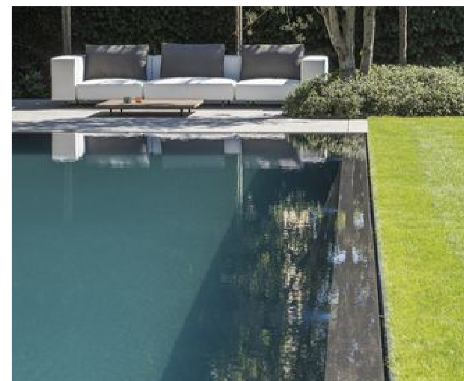
Granite pool tiling with flush wet edge coping
