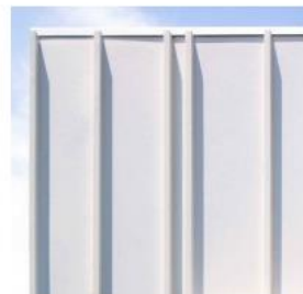
3. FC-01 Fibre-cement cladding & ceiling soffits
