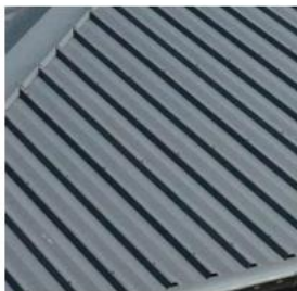
1. RS-01 Roof sheeting
