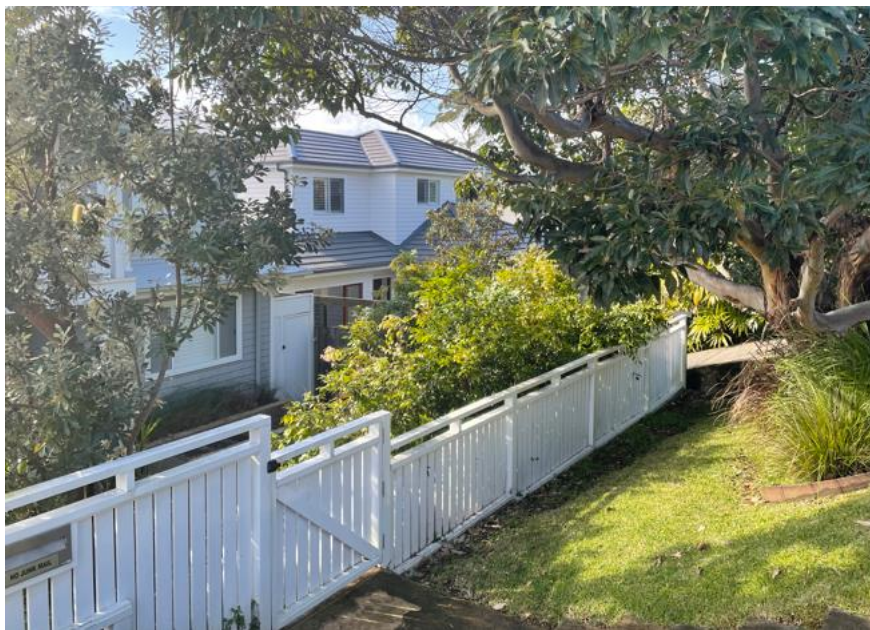
Figure 8. Front view of 59 Wyadra Road
