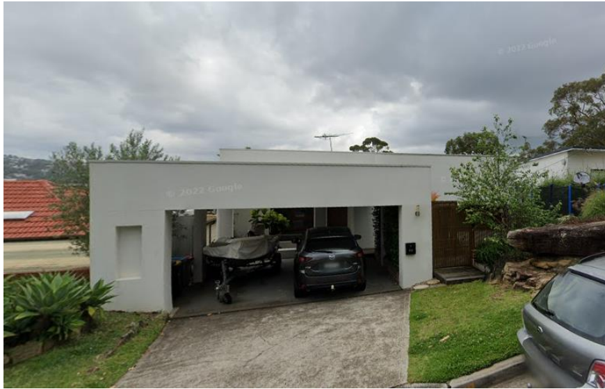
Figure 7. Double garage on nil setback at 69 Wyadra Ave
