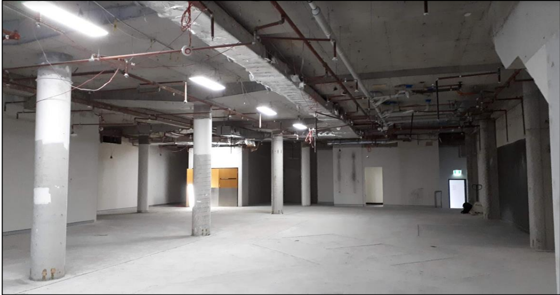
Figure 8. Existing internal ground floor facing south-east Source: Mecone
