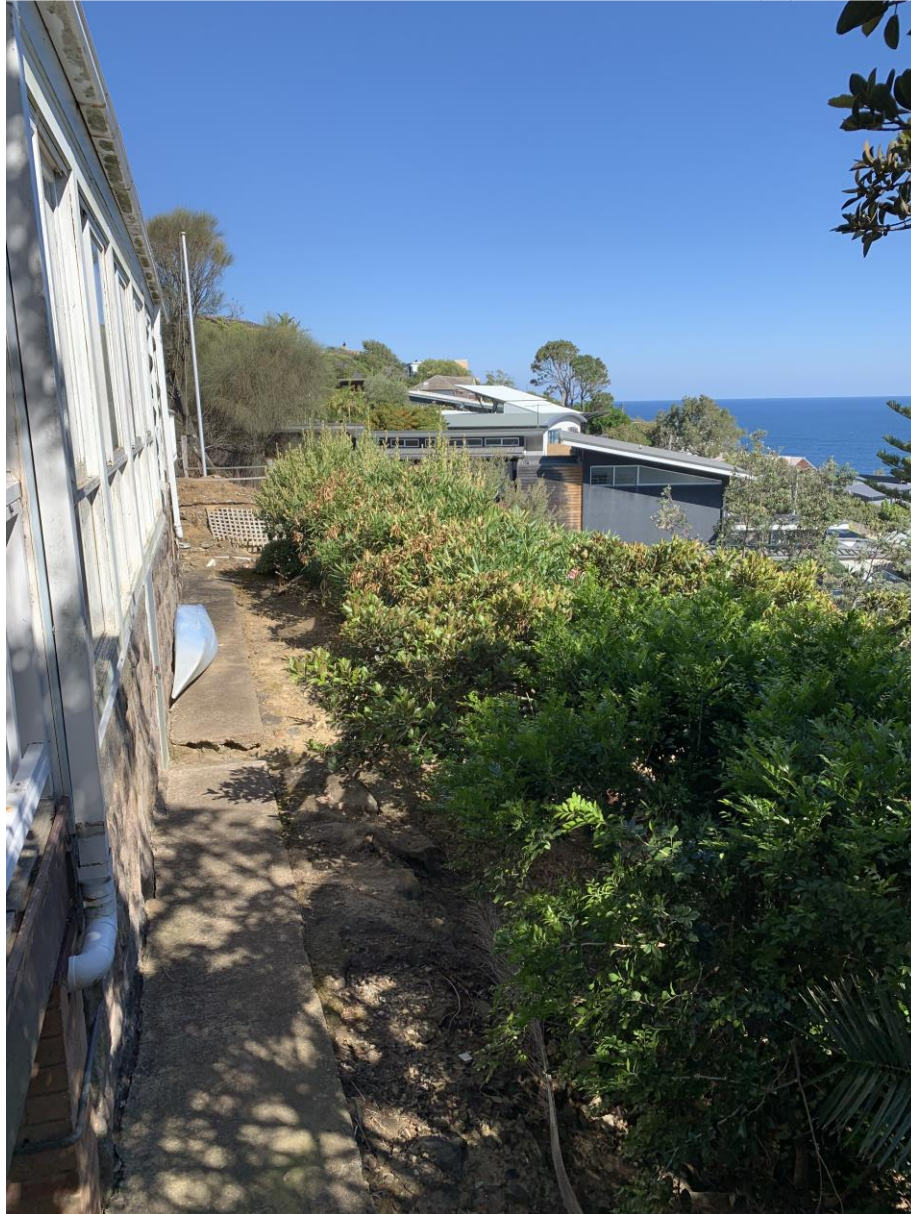
Fig 3: View looking east along the existing southern elevation of the dwelling
