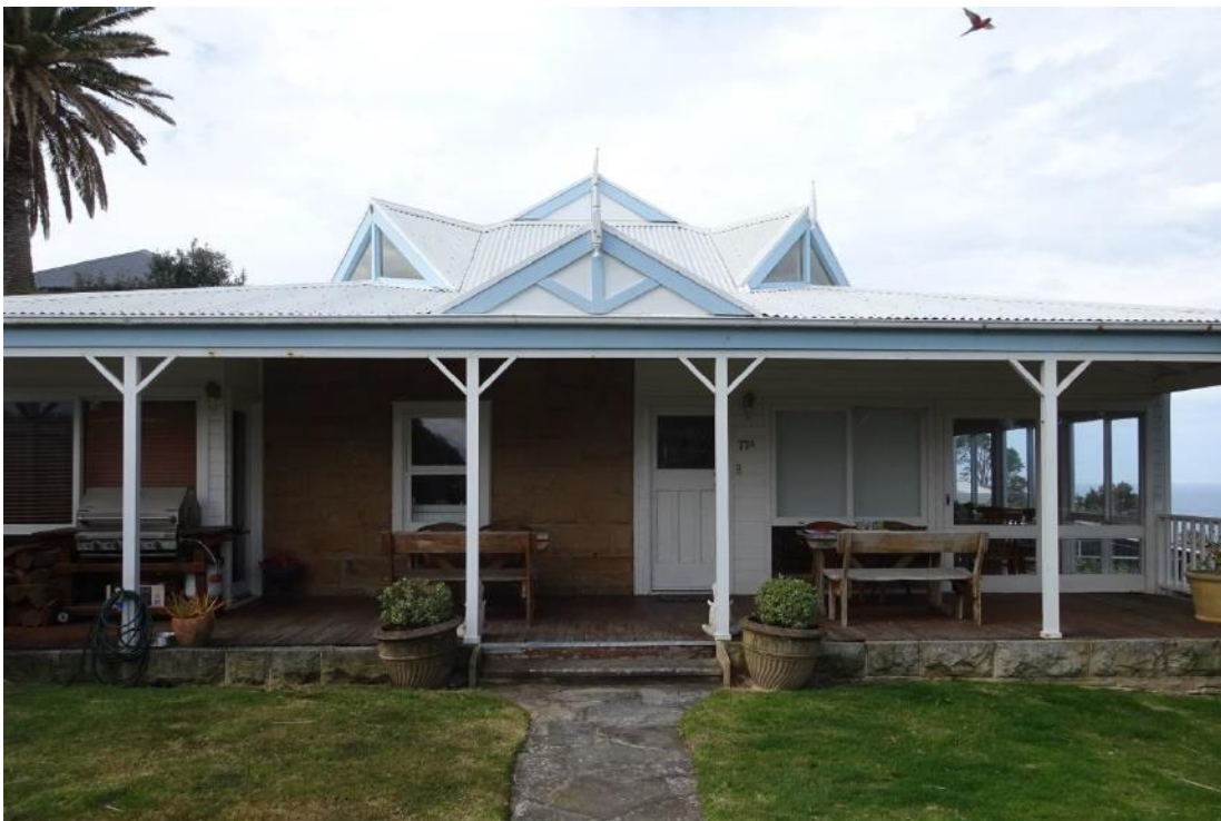
Fig 2: View of subject dwelling, looking south-east
