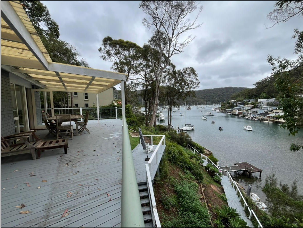
Photo 6: View to the west across the existing ground level deck showing the stairs and access path to the jetty and Browns Bay.
