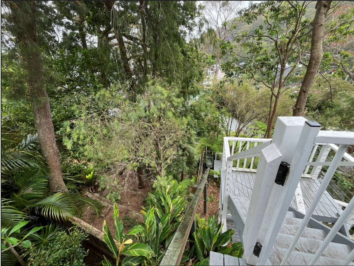
Photo 4: View to the north along the site's western side boundary showing the timber access stairs and inclinator.
