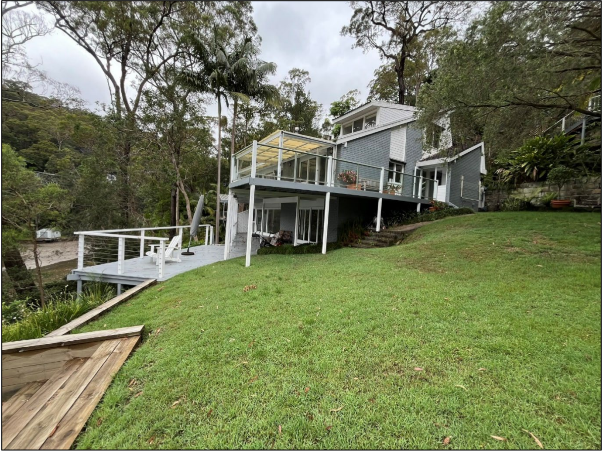
Photo 8: View of the dwelling from the top of the access stairs and pathway down to the waterfront.
