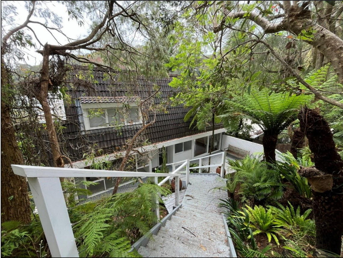
Photo 5: View of the rear of the existing dwelling from the top of the access stairs.
