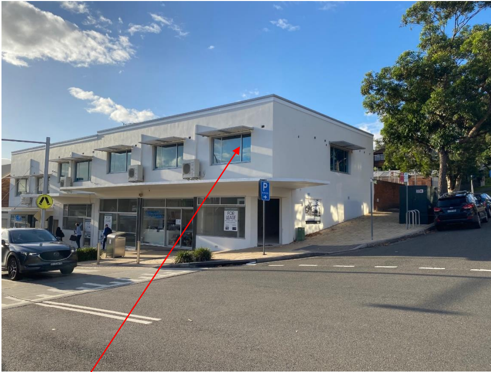
Subject premises – Level 1 / 28 Lawrence St
