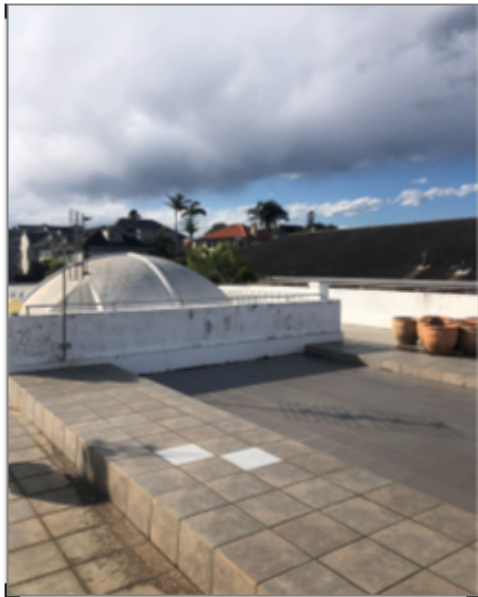
EXISTING ROOF TERRACE
