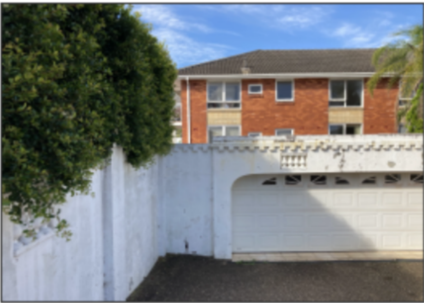
EXISTING GARAGE/ 30A ADDISON RD 8 BRUCE AVENUE UNITS BEHIND
