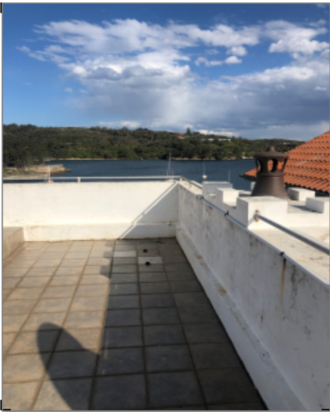
EXISTING ROOF TERRACE
