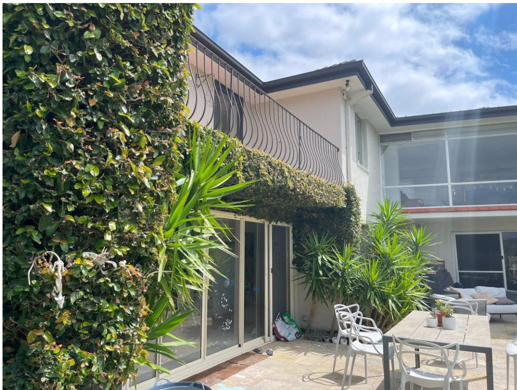
Fig 11: View of the rear, eastern elevation of the dwelling, looking north
