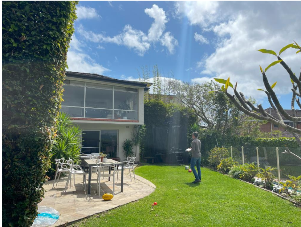
Fig 12: View of the rear, eastern elevation of the dwelling, looking north-east
