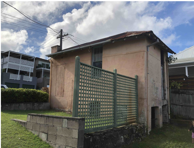
5 Rear view of garage
