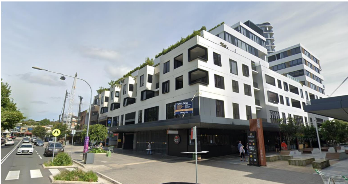
Figure 5 – Meriton Lighthouse development opposite subject site
