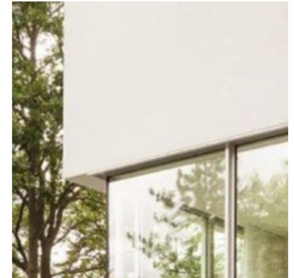
WD-01 - ALUMINIUM WINDOWS RB-01 - RENDERED CONCRETE BLOCK
