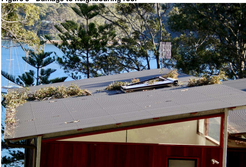
Figure 6 - Damage to Solar Panel
