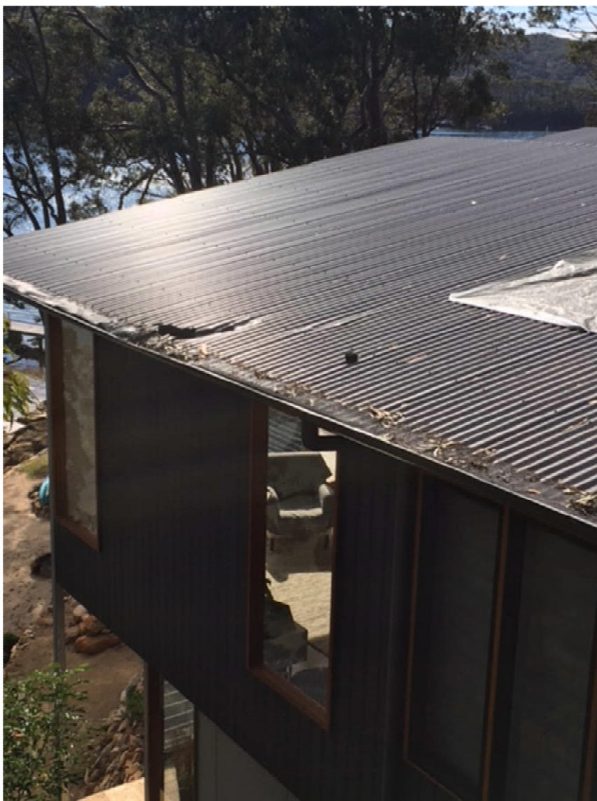
Figure 5 - Damage to neighbouring roof
