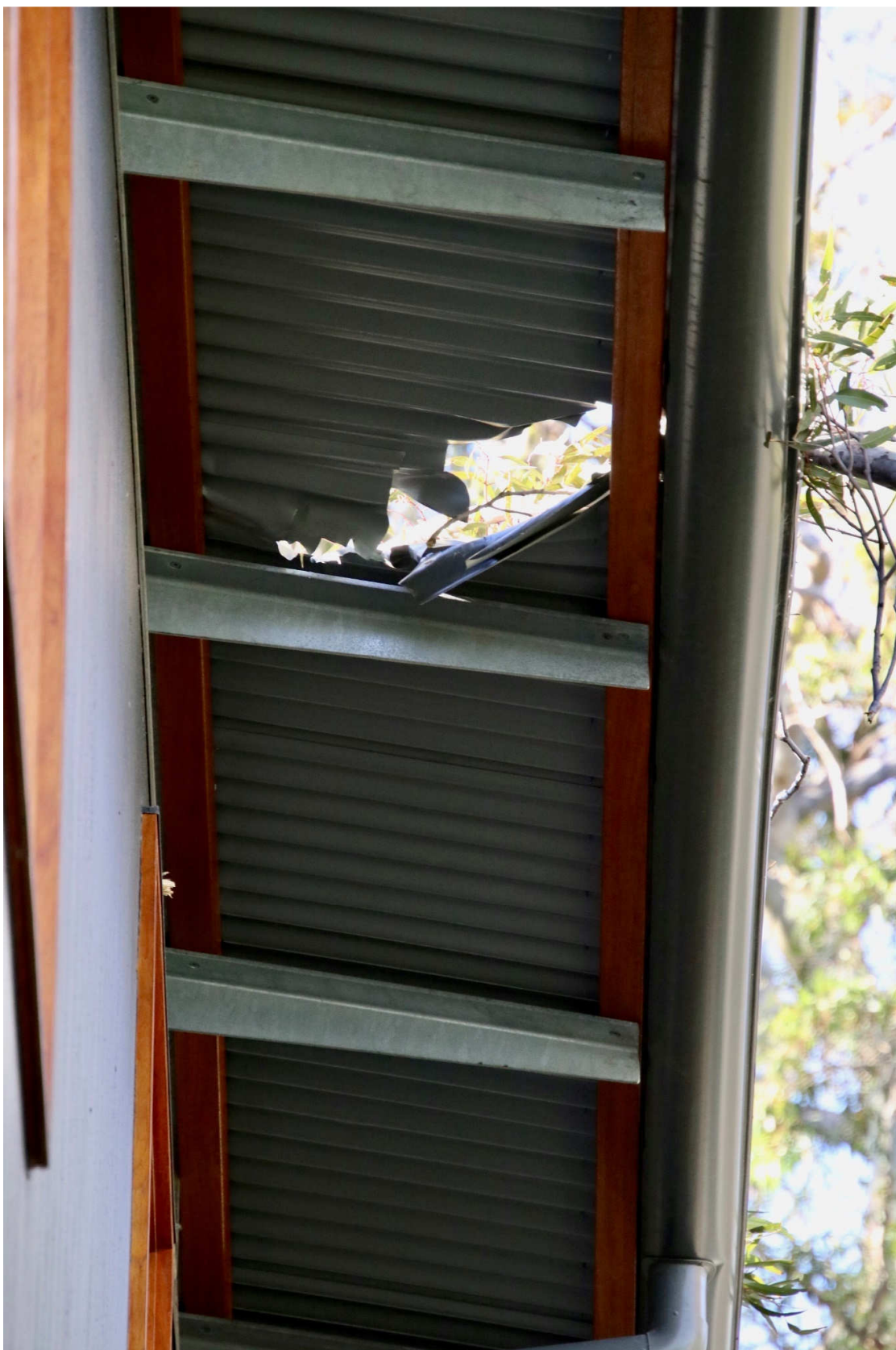
Figure 4 - Damage to neighbouring roof
