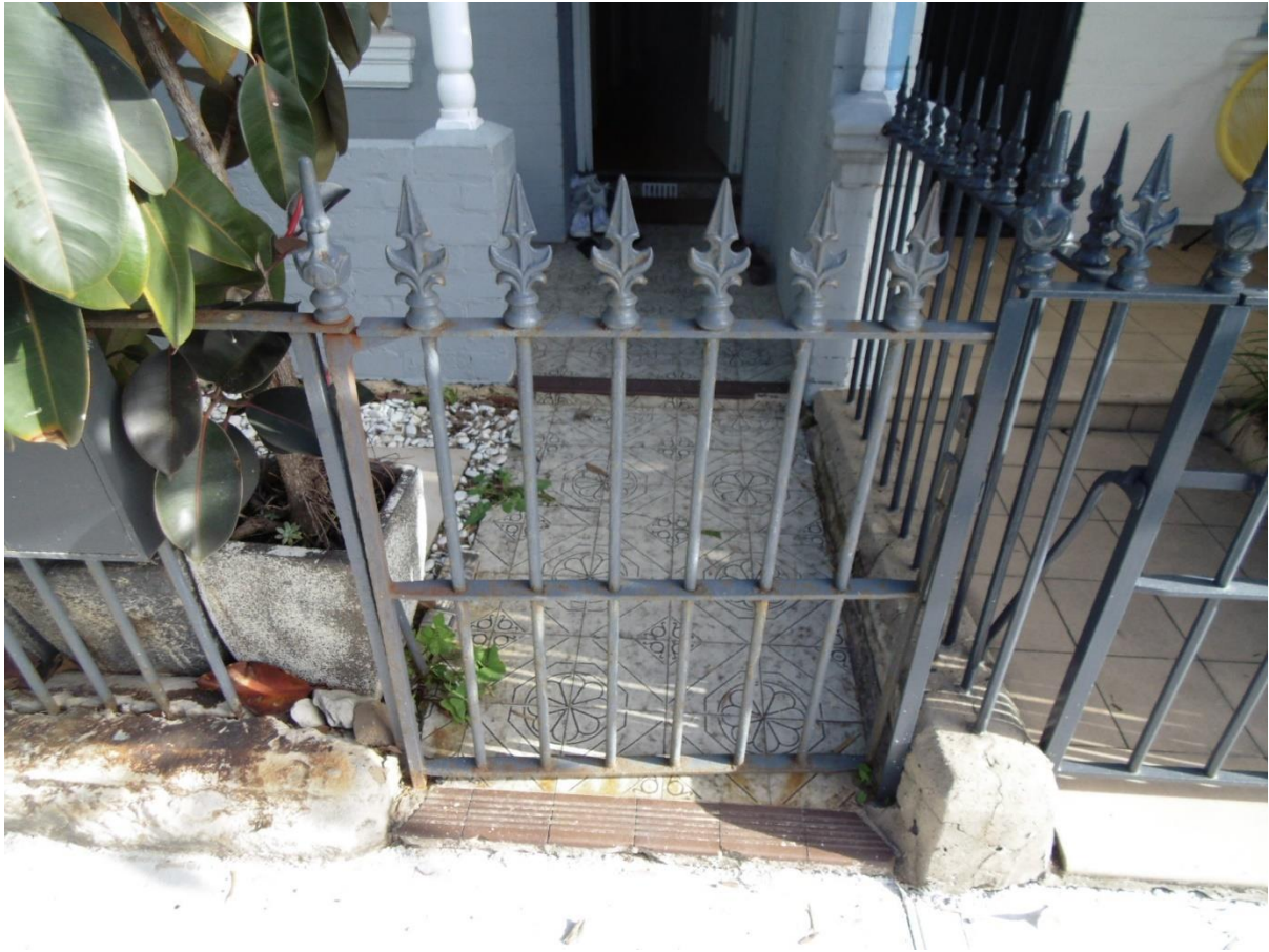
Front cast iron palisade gate
