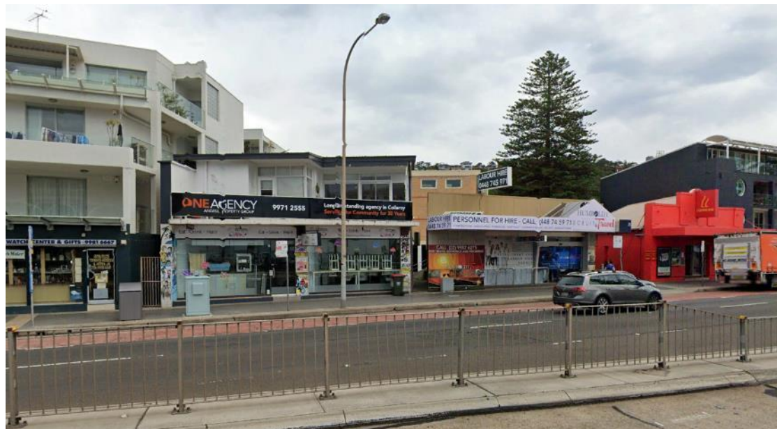
Figure 3 – Subject property as viewed from Pittwater Road
