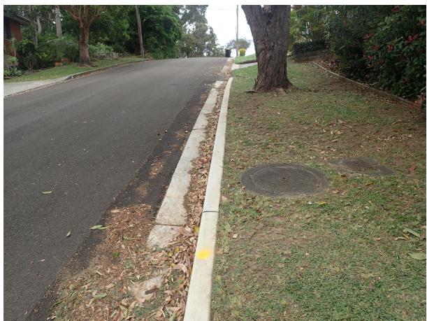
Plate 1 – T1 SW manhole and kerb renewal
