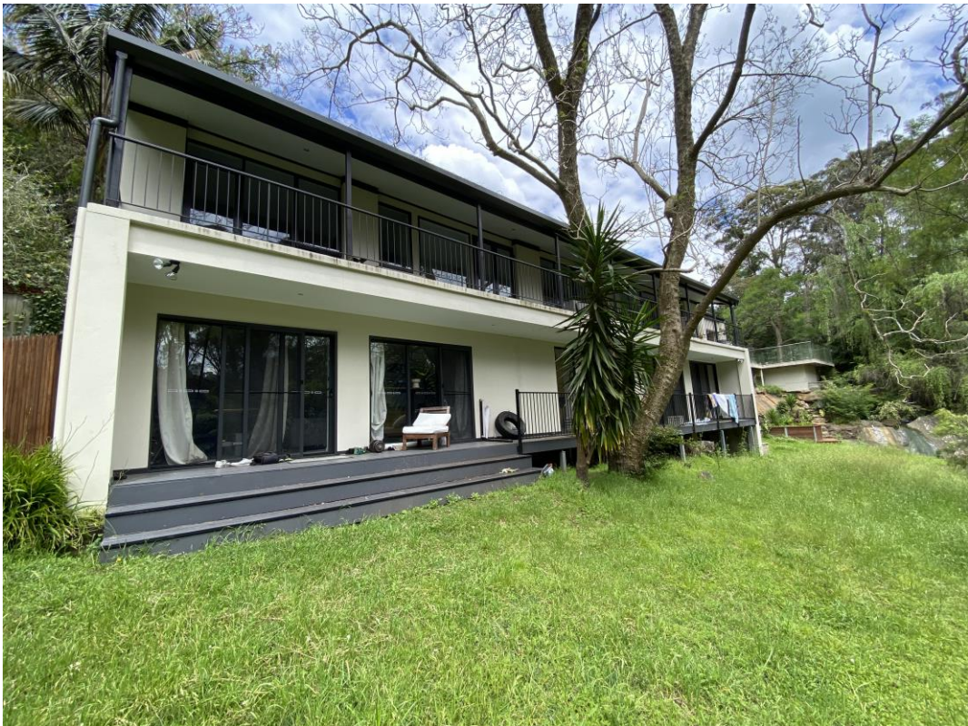
Figure 9. Looking south west, the rear of the existing dwelling
