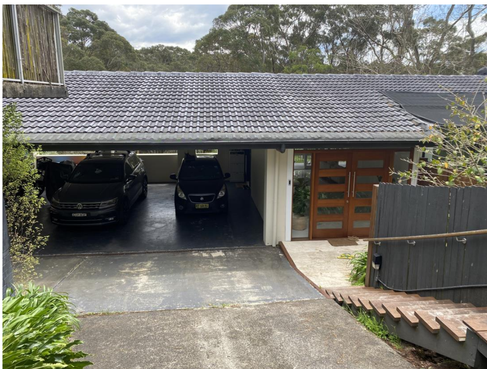
Figure 5. Looking north, the front entrance to the existing dwelling and the carport
