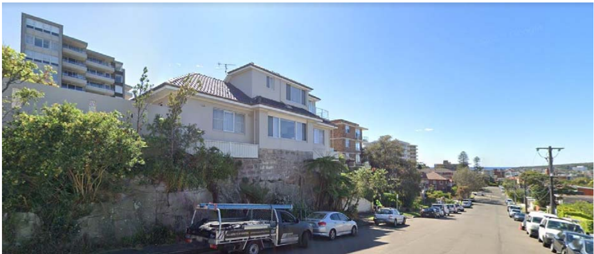
Fig 5. The existing streetscape on northern side of Fairlight St
