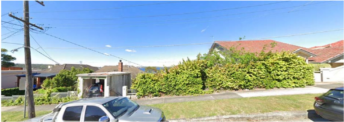
Fig 1. Existing site at 33-35 Fairlight St
