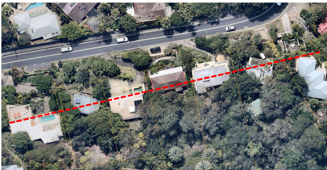
Figure 9 – Aerial image of Barrenjoey Rd with 10m front building line shown in the dashed red line Source: Nearmap and NBP
