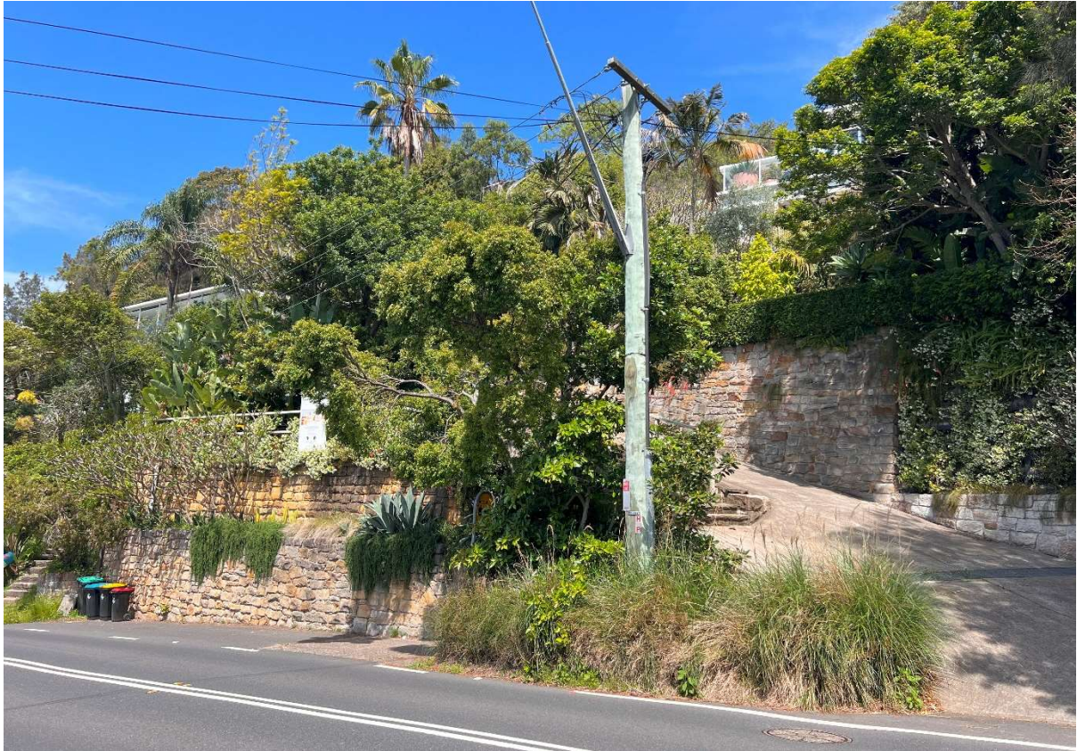
Figure 6 – Neighbouring dwelling to the west at 1162 Barrenjoey Road Source: NBP
