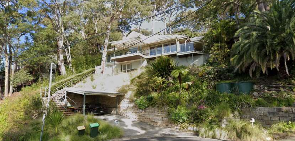
View of Subject site from Street
