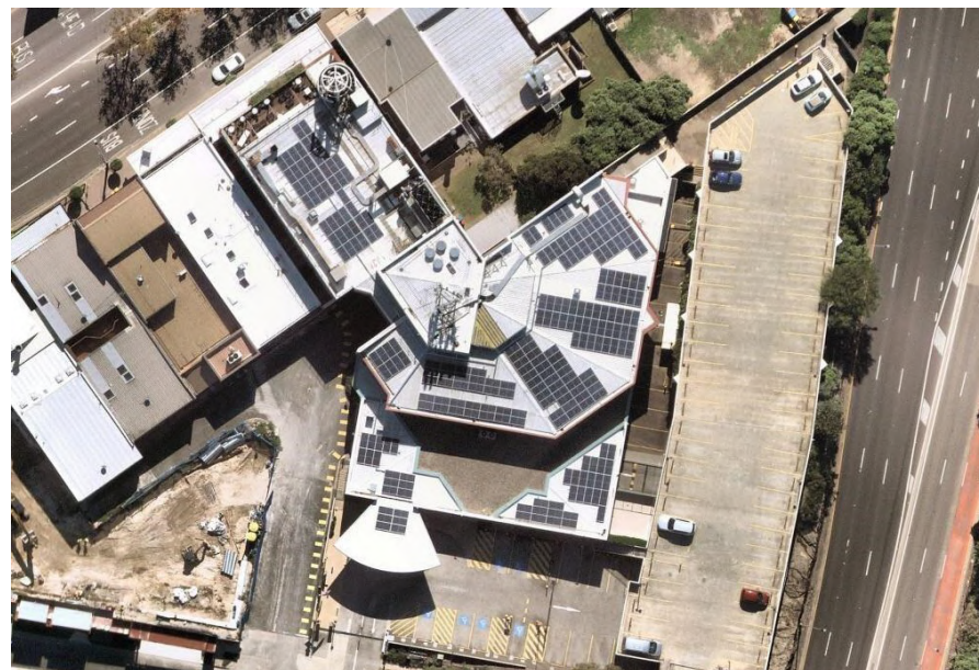
91kW PV array installed at Balgowlah RSL
