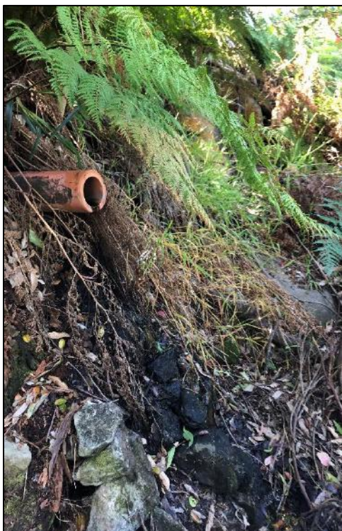
Photograph 6 and 7: View of stormwater pipe discharging onto slope below site (6) and adequate stormwater transfer away from site residence
