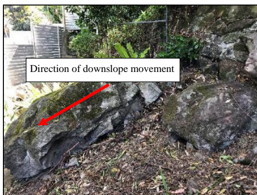
Photograph 4 and 5: View of the rear south of the site looking broadly north east at detached blocks apparently creeping downslope (4) and separation within mortared blocks
