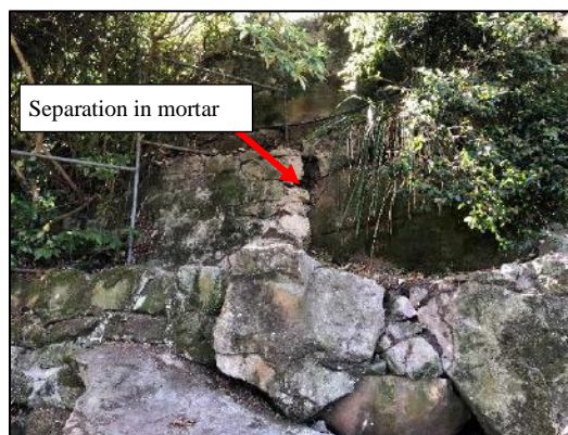
Photograph 4 and 5: View of the rear south of the site looking broadly north east at detached blocks apparently creeping downslope (4) and separation within mortared blocks
