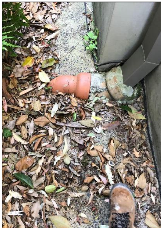
Photograph 6 and 7: View of stormwater pipe discharging onto slope below site (6) and adequate stormwater transfer away from site residence
