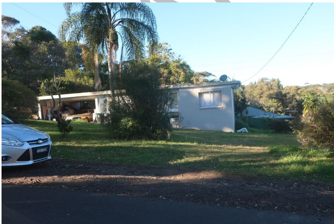
Figure 4.24 View of residential building on Lot 3 along The Avenue, facing south. AMAC Group IMG_7395 (21/06/2023).
