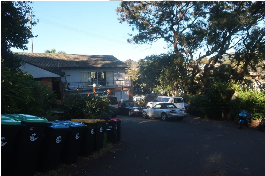
Figure 4.26 View of residential building on Lot 21 along The Avenue, facing south. AMAC Group IMG_7398 (21/06/2023).
