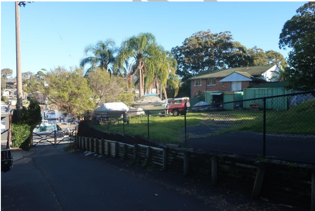
Figure 4.14 Lot 111 showing storage sheds and retaining walls, facing west. AMAC Group IMG_7404 (21/06/2023).
