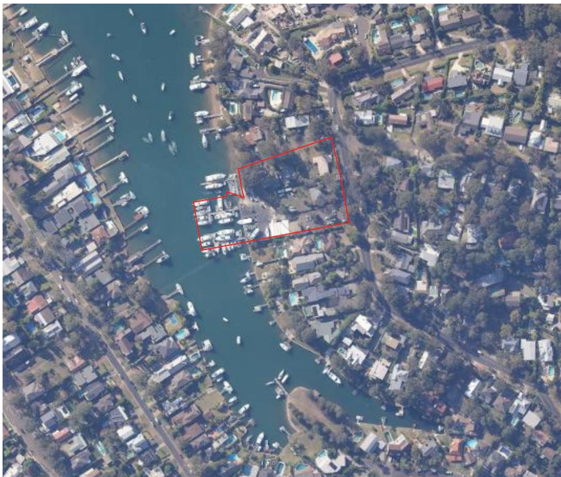
Figure 4.11 Current aerial photograph showing study site outlined in red. NSW Land Registry Services, Six Maps Viewer (accessed 3/07/23).
