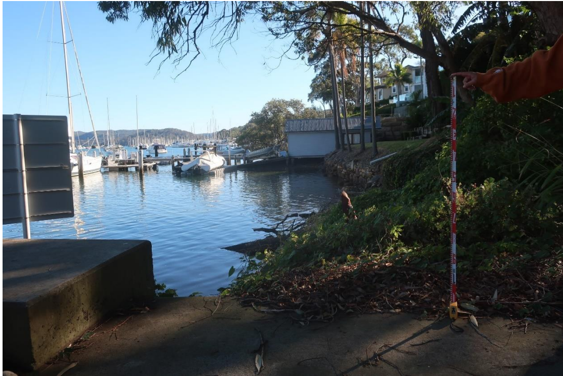
Figure 4.17 North edge of wharf showing shoreline, facing north. AMAC Group IMG_7417 (21/06/2023).
