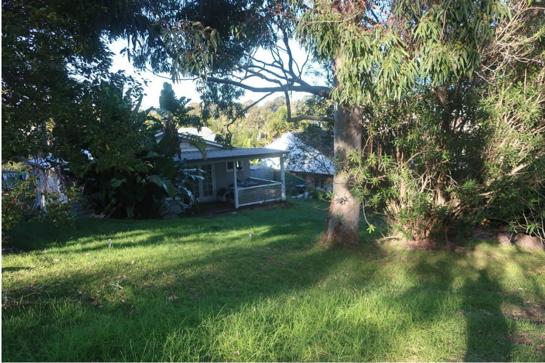
Figure 4.25 View of residential building on Lot 2 along The Avenue, facing south. AMAC Group IMG_7398 (21/06/2023).
