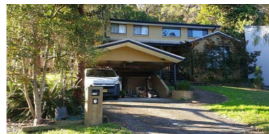
3. No. 6 Bellara Avenue , adjacent neighbour two storey dwelling
