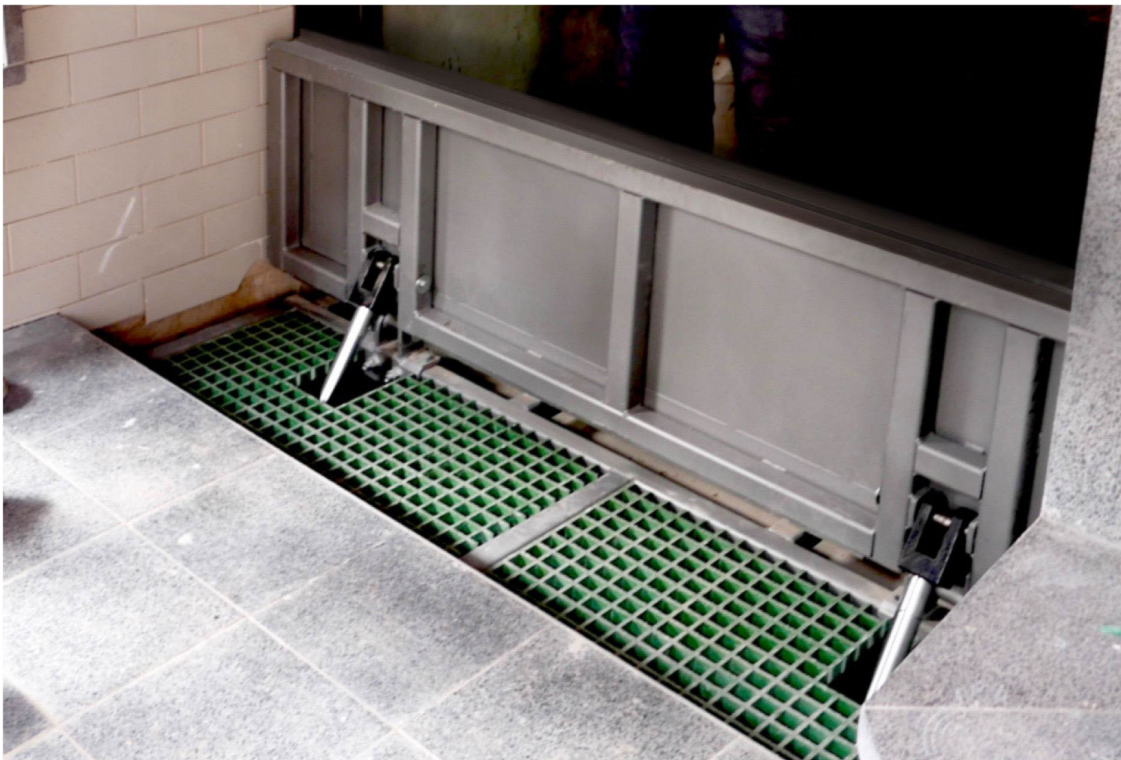
Figure 4 Self Closing Ram Push Flood Barrier Open Position - Courtesy of Flooding Solutions Pty Ltd
