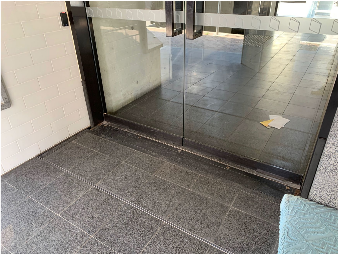
Figure 3 Self Closing Ram Push Flood Barrier Closed Position - Courtesy of Flooding Solutions Pty Ltd
