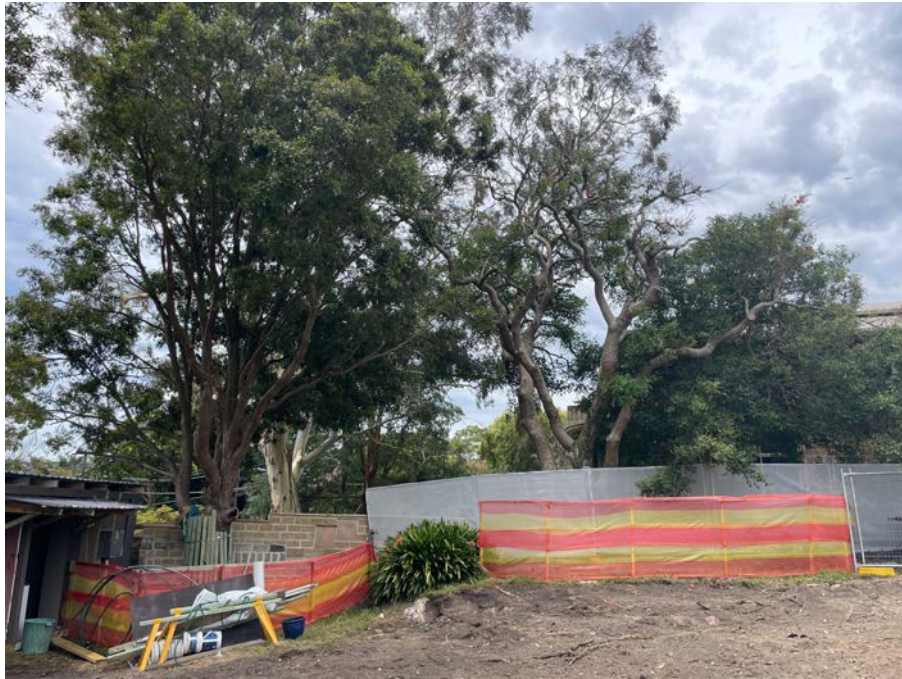
Photo 1: Tree 3 on left, inside site, and Trees 1 and 2 on right, inside neighbours. All 3 already have TPZ fencing installed and Tree 3 has trunk protection installed.
