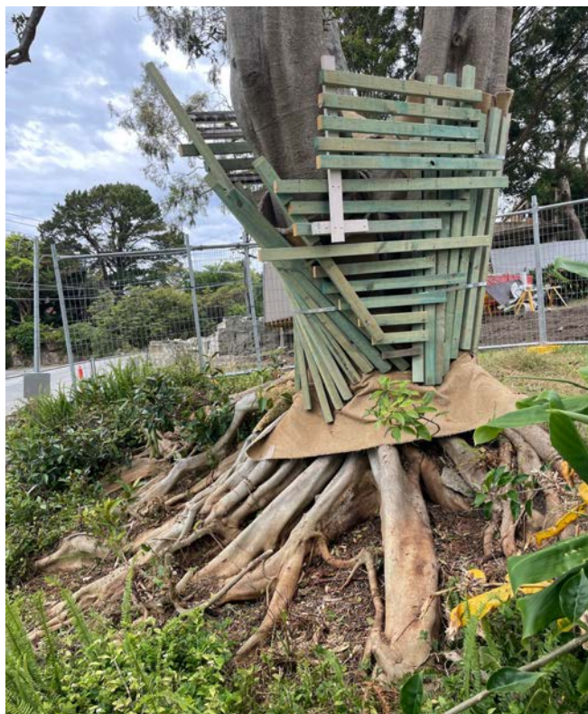
Photo 4: Tree 4 showing trunk protection and TPZ fencing installed already. Location of structural roots clearly visible
