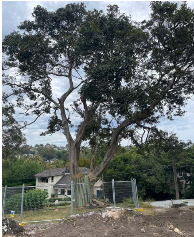
Photo 3: Tree 4 with TPZ fencing and trunk protection installed, Tree 5 behind at bottom of embankment.
