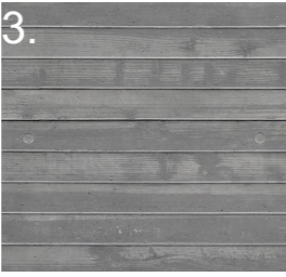
3. WALLS CONCRETE - OFF FORM
