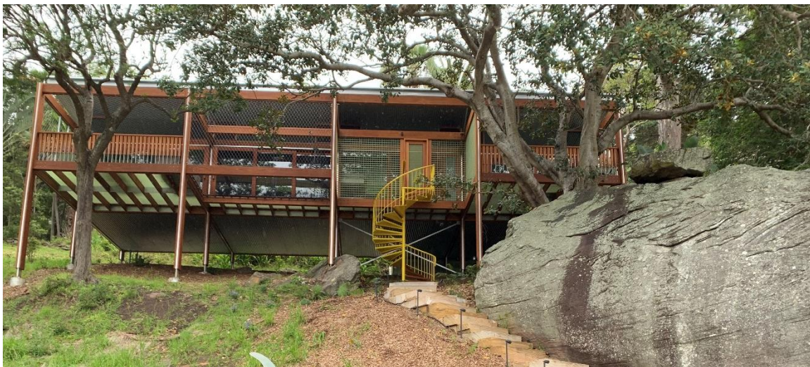
Photograph-12: Recently constructed dwelling within Lot 2, 1110 Barrenjoey Road, with large sandstone boulder and smaller detached unit on top, facing east
